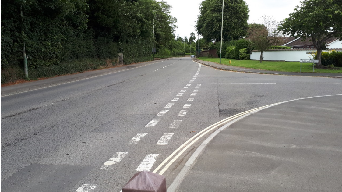
Photo 1 – Visibility from South side of crossing in an Easterly direction.
